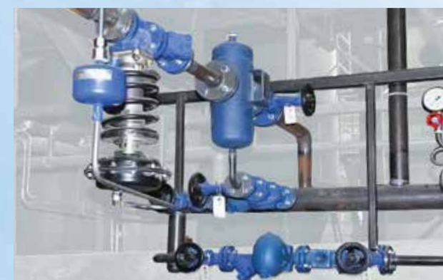
Steam pressure reduction. PREDU® with an upstream separator and ARI strainer
